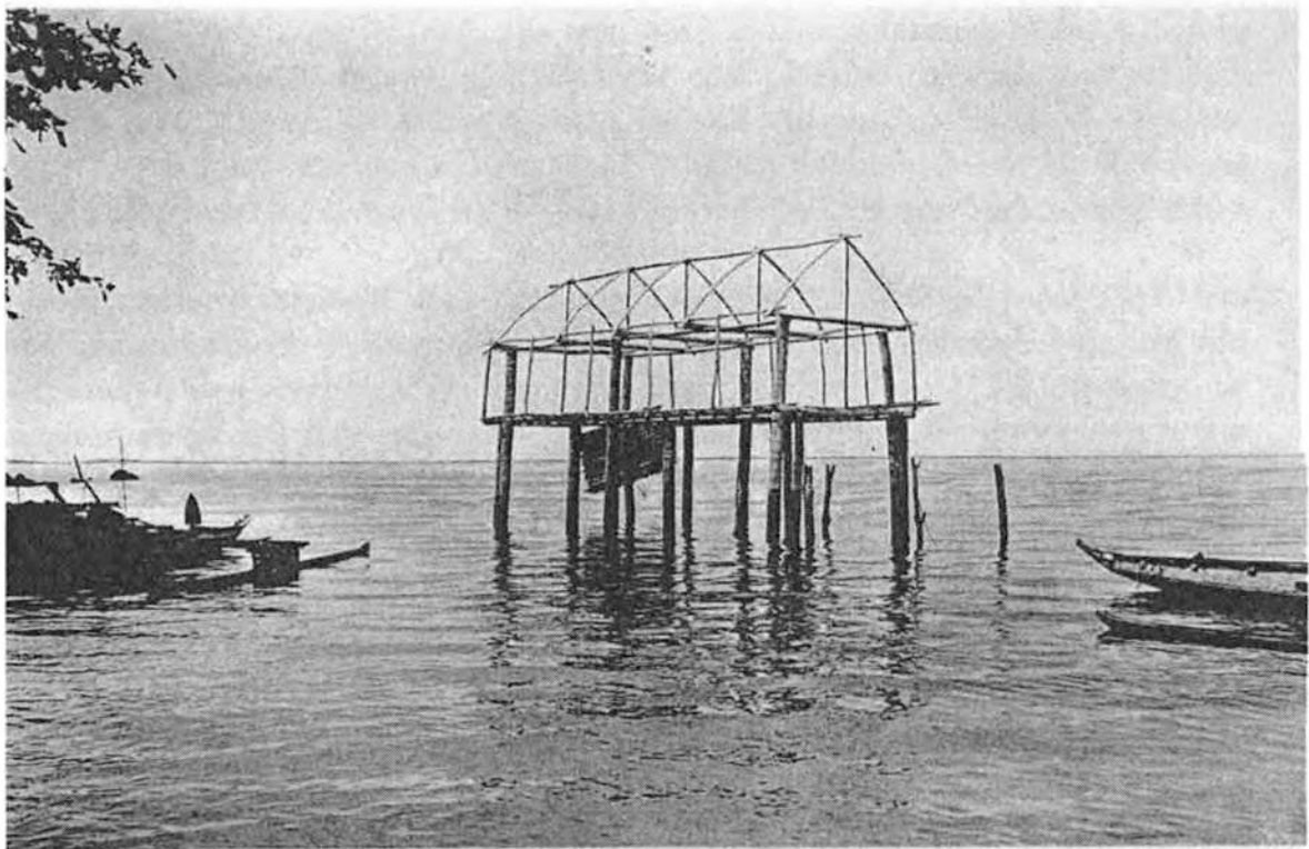
Framework of a pole building near Bird Island Bay
