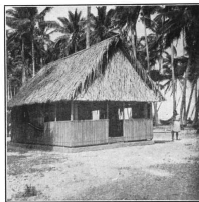
D. A house of the new style with concrete floor and walls of narrow wooden slats. This house won a prize in the house-building competition in 1934.
